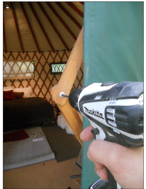
4. Rivets on elbows are removed.
