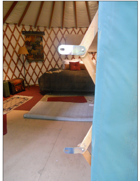
5. New hardware is bolted onto elbows.
