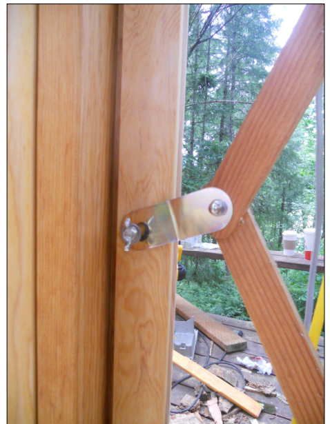
6. New hardware attaches to new door frame.
