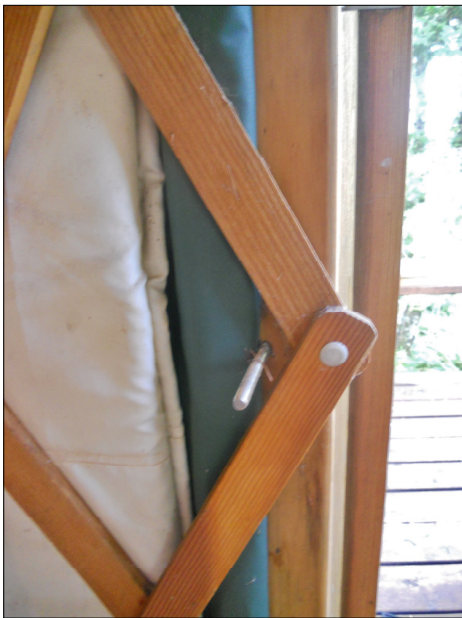
1. Old-style door frame attachment to lattice wall.
